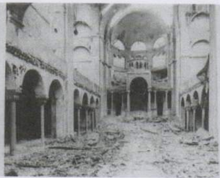
A badly damaged synagogue
